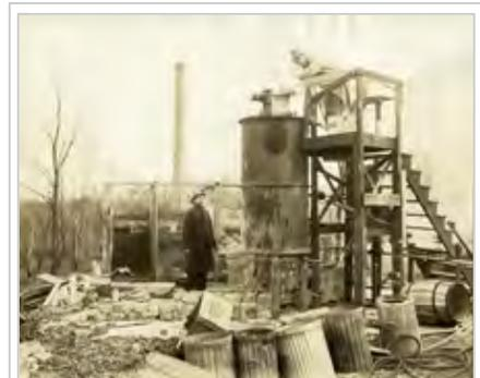
Charging the experimental blast furnace, Fixed Nitrogen Research Laboratory, 1930
