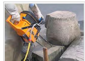
A chainsaw cutting concrete. The hose supplies cooling water.
