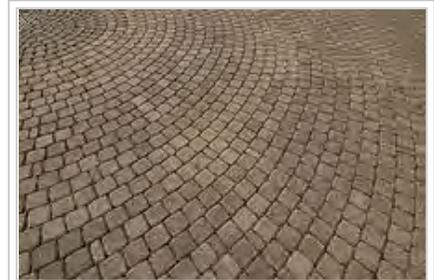
Regular concrete paving blocks
