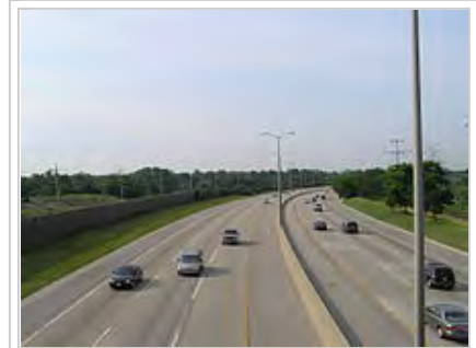
A highway paved with concrete.
