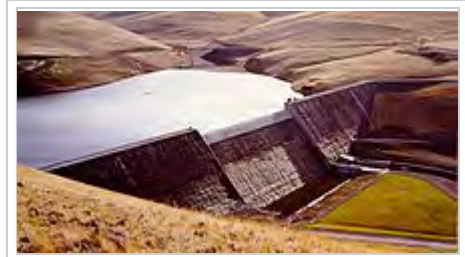
Willow Creek Dam, RCC gravity dam, Oregon, USA
