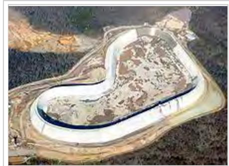
The rebuilt upper reservoir of the Taum Sauk plant, nearing completion in this photo, is the largest RCC dam in North America.<sup>[1]</sup>
