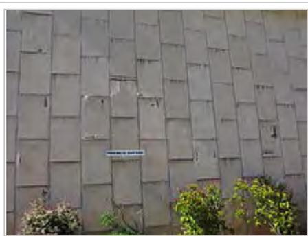
Concrete wall cracking as steel reinforcing corrodes and swells. Rust has a lower density than metal, so it expands as it forms, cracking the decorative cladding off the wall as well as damaging the structural concrete. The breakage of material from a surface is called *spalling*.
