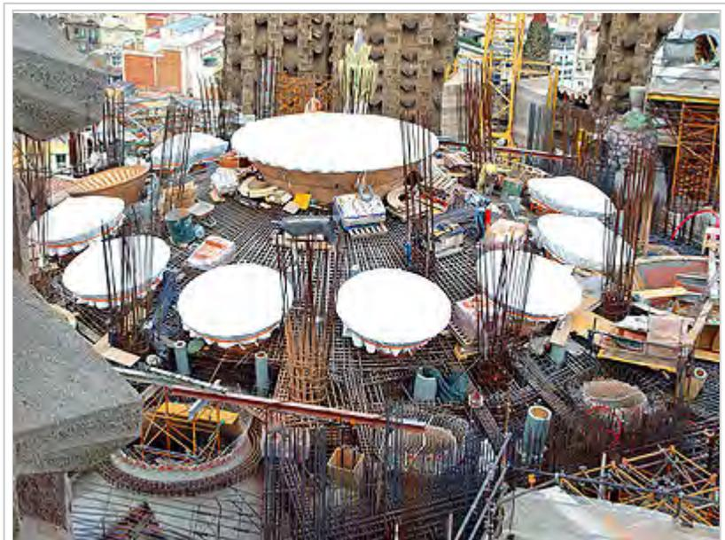
Rebars of Sagrada Família's roof in construction (2009)
