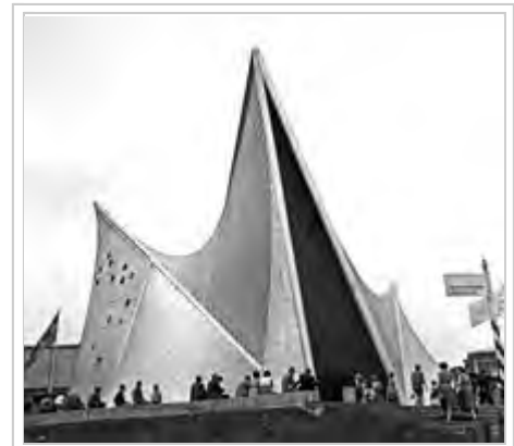
The novel shape of the Philips Pavilion was allowed by reinforced concrete.
