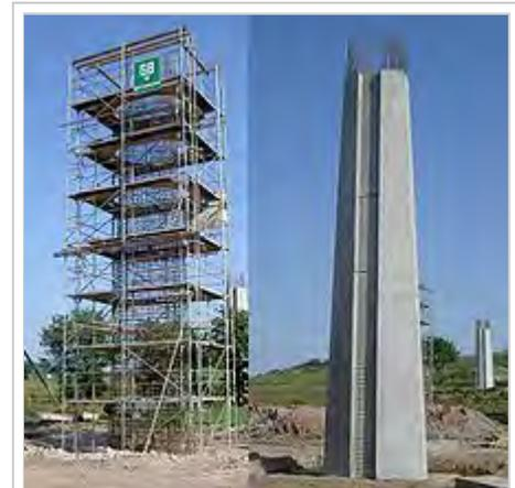
A heavy reinforced concrete column, seen before and after the concrete has been cast in place around the rebar cage.
