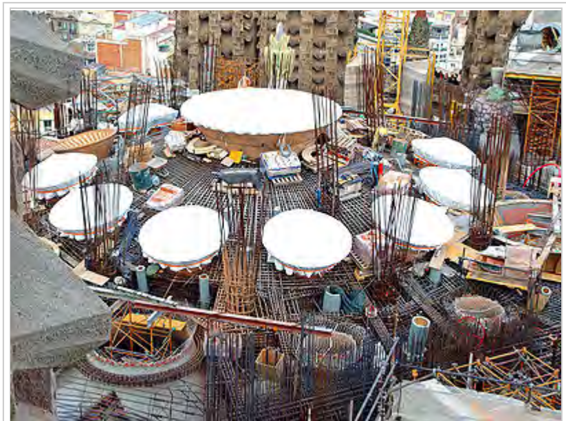
Rebars of Sagrada Família's roof in construction (2009)
