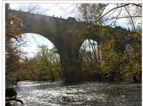
The Paulins Kill Viaduct, Hainesburg, New Jersey, is 115 feet (35 m) tall and 1,100 feet (335 m) long, and was heralded as the largest reinforced concrete structure in the world when it was completed in 1910 as part of the Lackawanna Cut-Off rail line project. The Lackawanna Railroad was a pioneer in the use of reinforced concrete.
