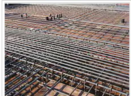
Rebar constructed to properly reinforce a beam element, awaiting concrete to be poured.
