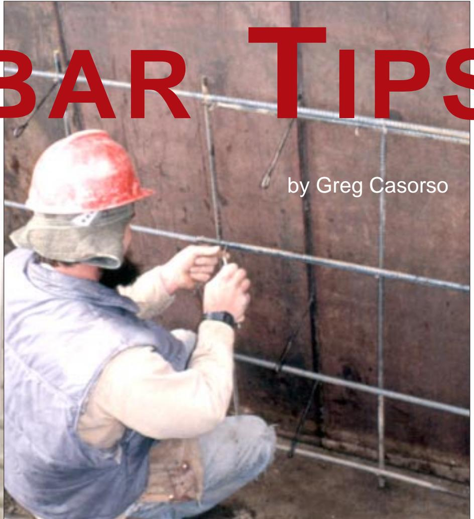
Reinforcing steel enables concrete to resist bending forces — but you have to place it and tie it correctly
