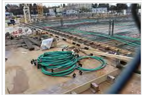
Unbonded slab post-tensioning. Installed strands and edge-anchors are visible, along with prefabricated coiled strands for the next pour
