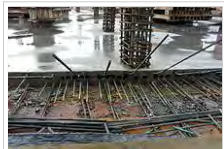
Unbonded slab post-tensioning. End-view of slab after stripping, showing individual strands and stressing-anchor recesses
