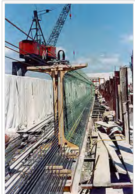
Pre-tensioned bridge girder in precasting bed. Note single-strand tendons exiting through formwork
