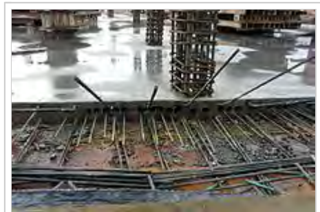
Unbonded slab post-tensioning. End-view of slab after stripping, showing individual strands and stressing-anchor recesses
