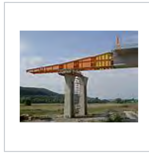
Autobahn A73 Itz Valley, Germany
