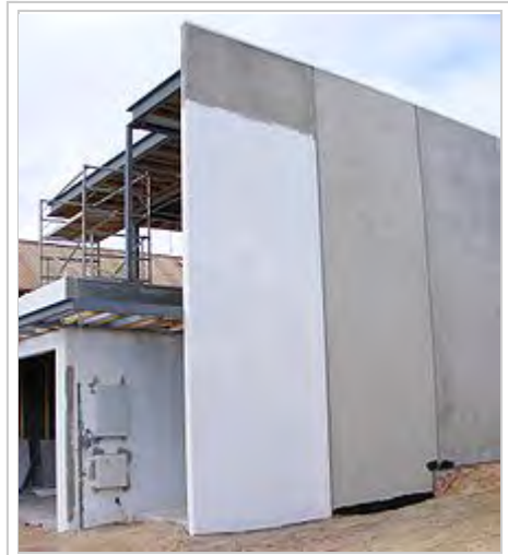
A precast concrete walled house under construction
