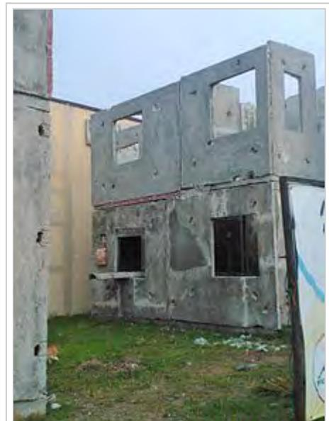
An example of low-quality precast concrete with exposed dowels, connectors and presence of cracks and malformations even during its installation.
