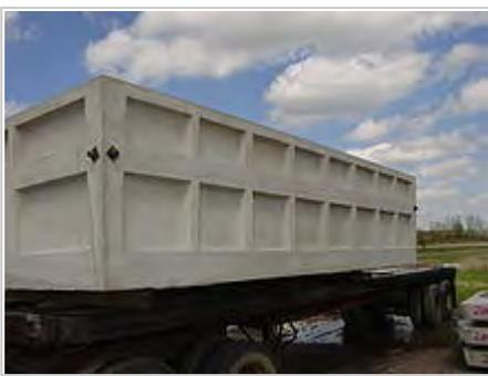
A precast concrete hazardous material storage container.
