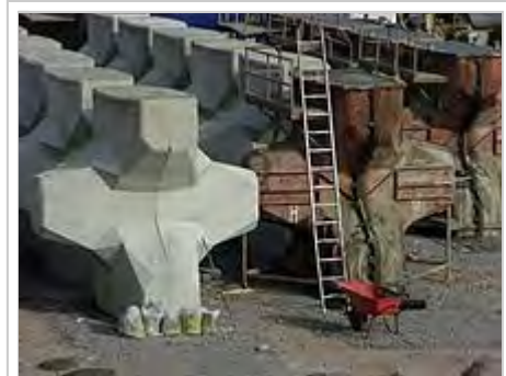
A precast concrete armour unit (ACROPODE).
