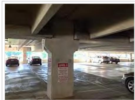
Precast parking structure showing an interior column, girders and double-tee structural floors. The two gray circles are covers to close the lifting anchor holes.
