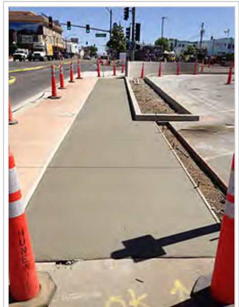
Freshly laid concrete
