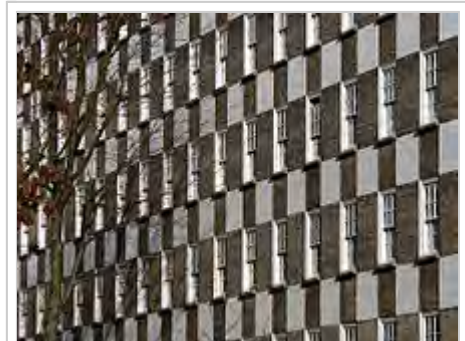
Decorative use of Portland cement panels on London's Grosvenor estate
