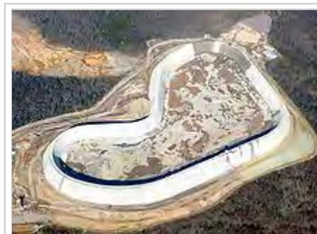
The upper reservoir of Ameren's Taum Sauk hydroelectric plant was constructed of roller-compacted concrete that included fly ash from one of Ameren's coal plants.<sup>[27]</sup>
