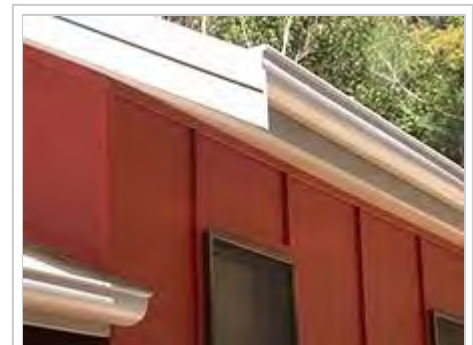
Detail - timber battens on fiber cement cladding, dwelling addition, Hardys Bay, NSW, Australia
