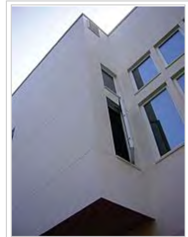
HardiePlank on design-build addition, Ithaca NY
