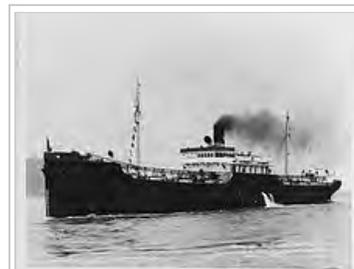
The American concrete oil tanker *Palo Alto*, originally meant for merchant service in the first World War, but completed in 1919. (Naval History and Heritage Command - Photo NH 799)
