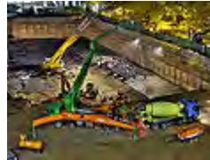
Photo showing a concrete pump working a large foundation pour, showing deployed outriggers, rebar mats, and concrete mixer delivering concrete.
