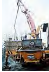
A Putzmeister concrete pump in Germany in 1985
