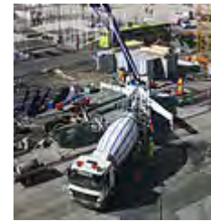
Fully deployed concrete pump, showing outriggers and boom in use while receiving concrete.
