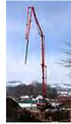
Boom concrete pump
