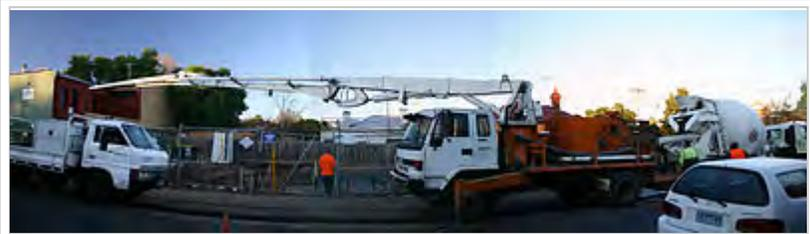
Because it is a fluid, concrete can be pumped to where it is needed. Here, a concrete transport truck is feeding concrete to a concrete pumper, which is pumping it to where a slab is being poured.
