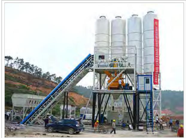
In this photo, you can see a set of belt conveyor concrete plant being installed. It clearly shows the belt conveyor concrete plant's main structure, batch hopper, belt conveyor, cement bins, mixer, etc.
