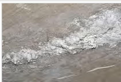
Example of secondary efflorescence in parking garage exposed to diluted road salt from vehicles entering the garage during winter.
