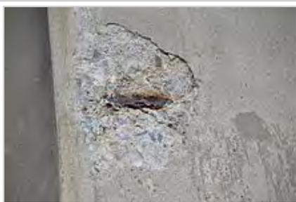
Example of flat piece of concrete having dislodged with corroded rebar underneath, Welland River bridge across Queen Elizabeth Way in Niagara Falls, Ontario.
