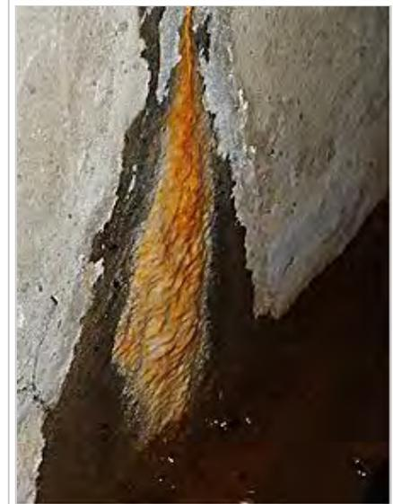
Calthemite flowstone stained orange from rusting reinforcing (iron oxide) being deposited along with calcium carbonate
