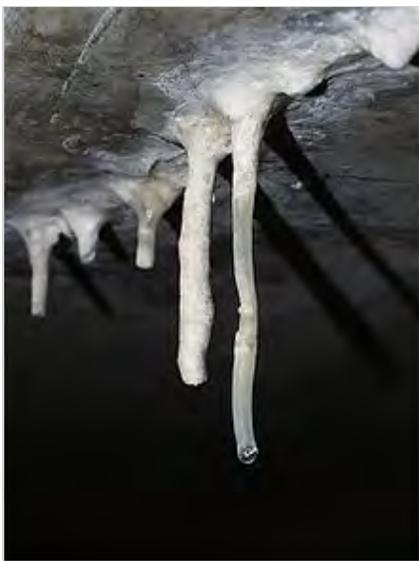
Stalactites growing beneath a concrete structure as a result of calcium hydroxide being leached from concrete and deposited as calcium carbonate to create calthemite forms beneath structure
