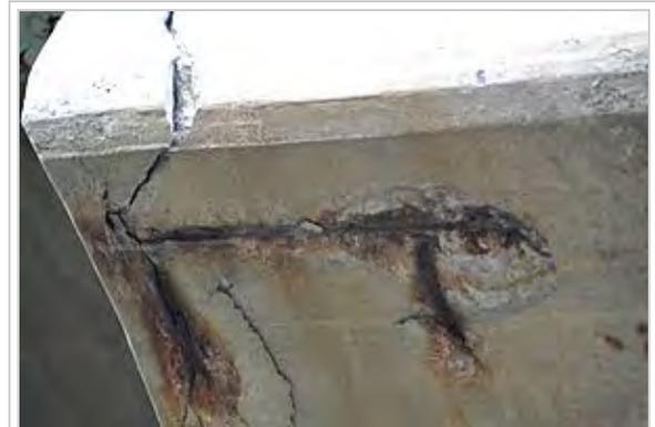
Degraded concrete and rusted, exposed rebar on Welland River bridge of the Queen Elizabeth Way in Niagara Falls, Ontario.
