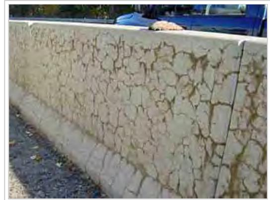
Typical crack pattern associated to the alkali-silica reaction affecting a concrete step barrier on a US motorway (photograph, courtesy of the Federal Highway Administration (US Department of Transportation).
