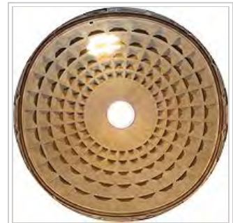
Interior of the Pantheon dome, seen from beneath. The concrete for the coffered dome was laid on moulds, probably mounted on temporary scaffolding.
