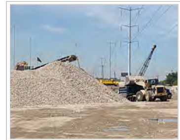
Recycled crushed concrete, to be reused as granular fill, is loaded into a semi-dump truck.
