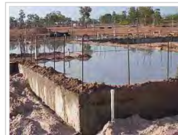
A concrete slab ponded while curing.
