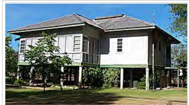
A pre-WW2 house in Darwin. The roof is sheeted with corrugated fibro sheets and the walls with flat fibro sheeting, with fibro battens covering the joints.
