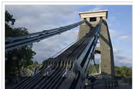
Eyebar chain cables of Clifton Suspension Bridge
