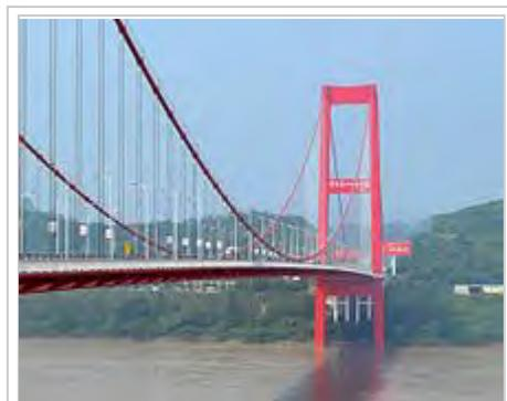
The Yichang Bridge, a plate deck suspension bridge, over the Yangtze River in China
