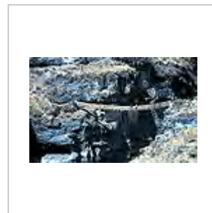
The new bridge is now complete and in use.
