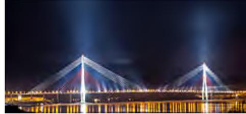
The Russky Bridge's central span measures 1104 meters. It is the world's longest cable-stayed bridge.
