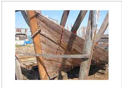
Plank fixing, trenails and red lead paint, Quy Nhon.
