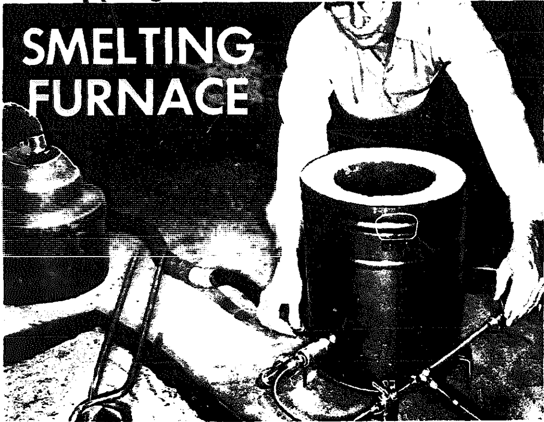
ADJUSTING FLAME. Burners have separate gas valves for delicate flame adjustment. Single valve controls air supply. Sheet-metal box containing dry sand on which the molding flask is set, is placed near furnace
