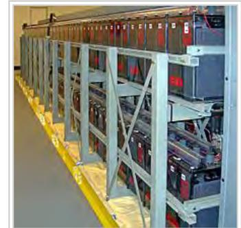
A battery bank used for an uninterruptible power supply in a data center
