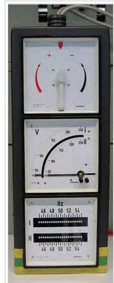
From top to bottom: synchroscope, voltmeter, frequency meter. When the two systems are synchronized, the pointer on the synchroscope is stationary and points straight up.
