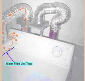
Dryer Diverter Slide Switch Shown In Heat Recovery Position
