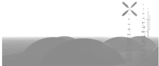
economical it is in this regard. This shape can enclose the maximum amount of space with the least surface area, but any concrete used in the building must be reinforced to prevent collapse. Another virtue-and key, as far as we are concerned-is the suitability of such a building for hydroponics. The viability of hydroponics is dependent upon an ability to control energy costs, and the dome structure is ideal in this respect.
